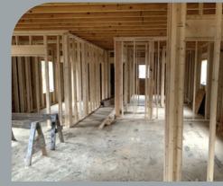
North Main Ave. before
